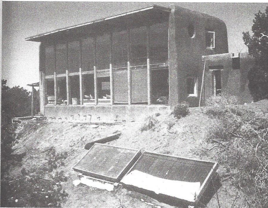
Figure 25.8. Wright's pioneering passive solar house, built in 1972. The auxiliary heating system in the foreground were made unnecessary by the passive design and materials.
